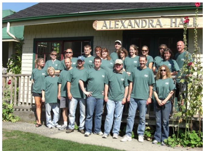
KNV's Partners and Managers volunteering a day to work at Camp Alexandra doing repairs.
